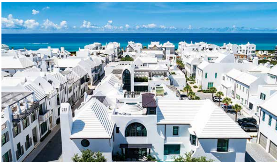
Alys Beach is known for its iconic white architecture, carefully designed streetscapes, and commitment to architectural integrity along Walton County's Scenic Highway 30A corridor.
