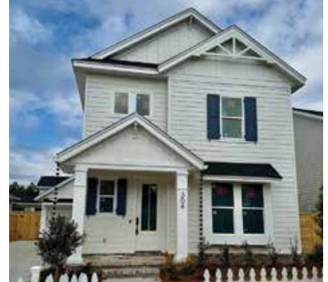
304 GAZELLE COURT 4 Bedroom | 2.5 Bath | 2,026 SF $601,000 | completed February 2026 Listed by Kelly Shephard 850.543.7353
